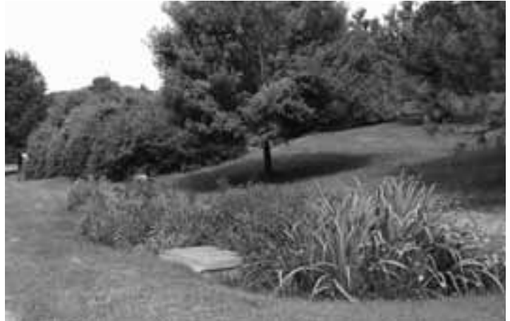
MDA worked with the South River Federation to install three rain garden/bioretention areas on the grounds that are helping to capture and filter stormwater and non-point source runoff that flows into Broad Creek and the South River.
